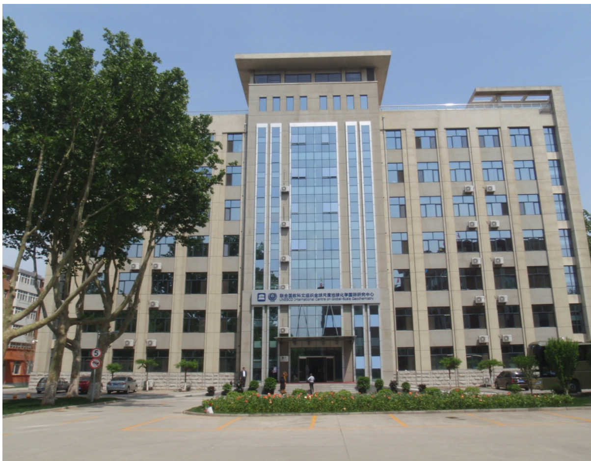
Figure 36. Building of the UNESCO International Centre on Global-scale Geochemistry, Langfang, P.R. China.
